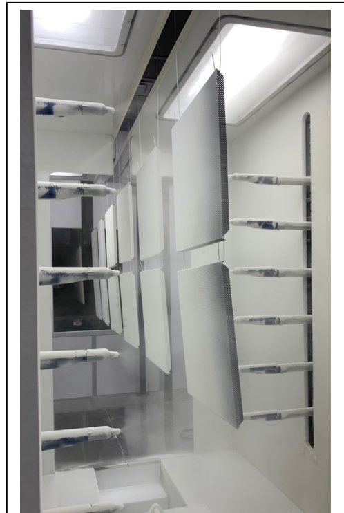
Gordon Inc.'s new application booth showing reciprocating guns applying an architectural powder coating on both sides of ceiling panels.
